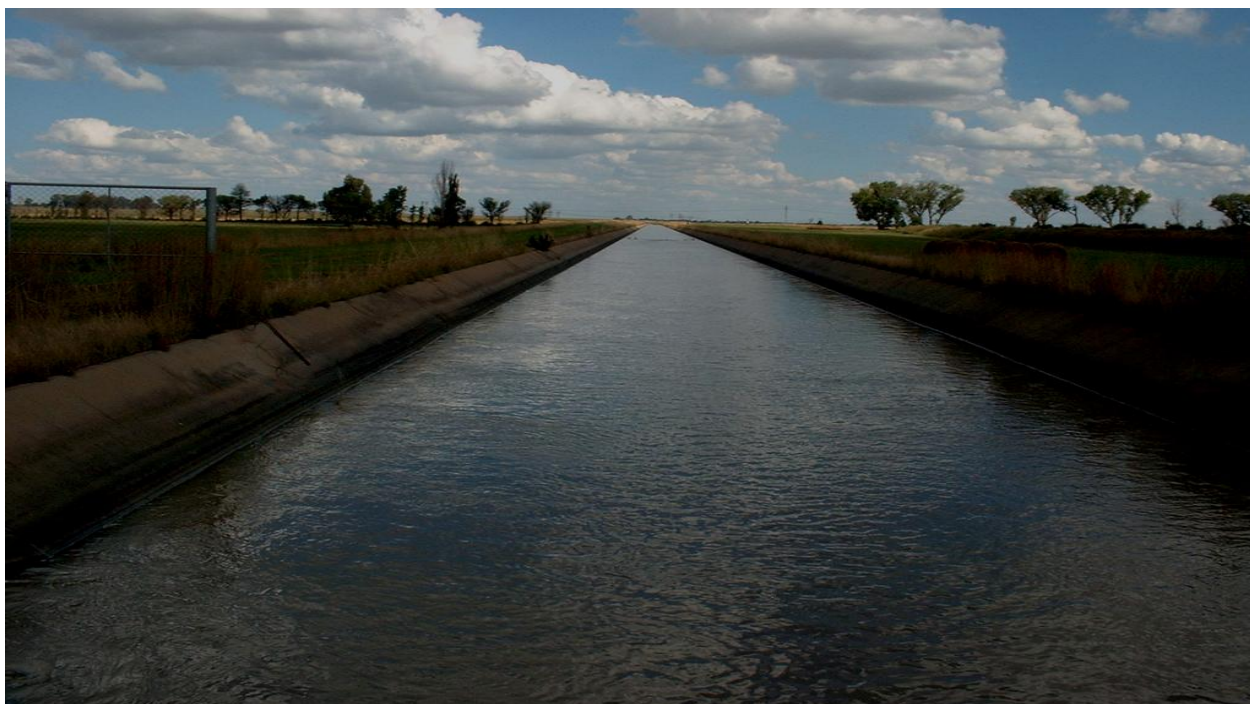
Figure 3.2: The open canal system transporting water from the Vaal Dam to the ZWTP where the water undergoes a series of purification processes.
