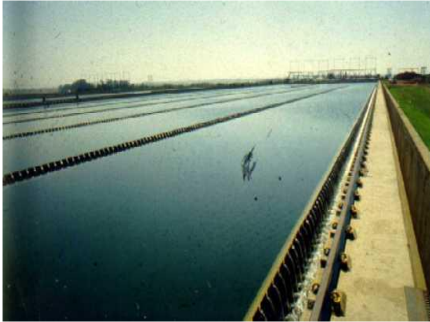
Figure 4.2: Sedimentation tanks of Rand Water's Zuikerbosch treatment plant close to Vereeniging (Google earth). Samples before filtration were collected at this locality in the treatment plant.
