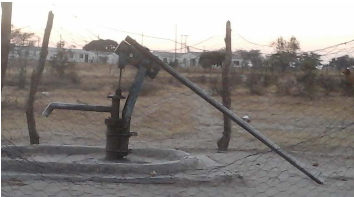
Image 4.3: Borehole water source in Chivi District: servicing both the local school and the community
