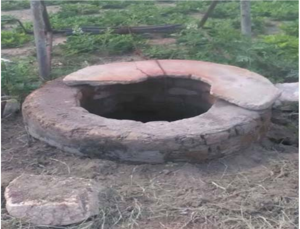
Image 4.5: Unprotected compound shallow well used for domestic consumption
