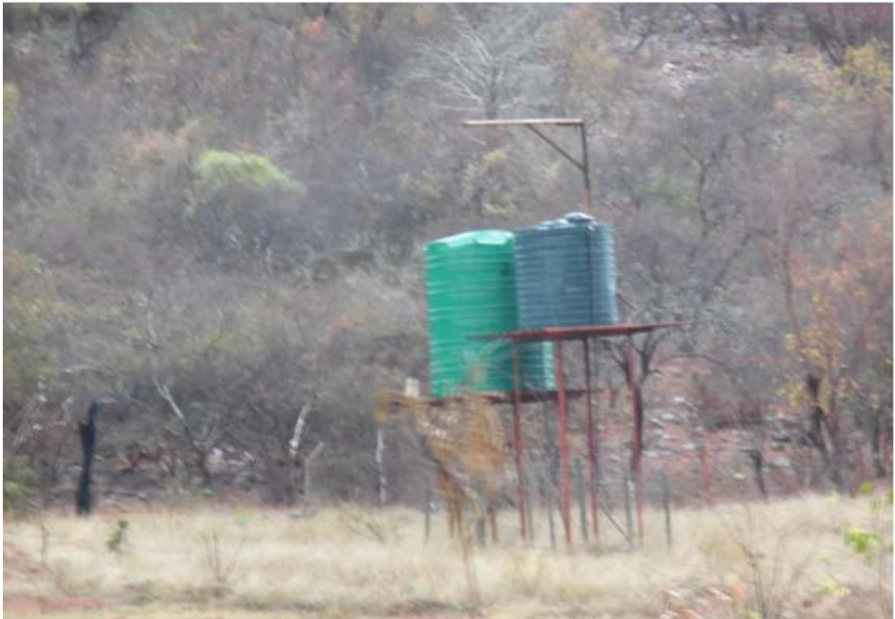
Image 5.5: Jojo tanks used for storing water from personal boreholes.
