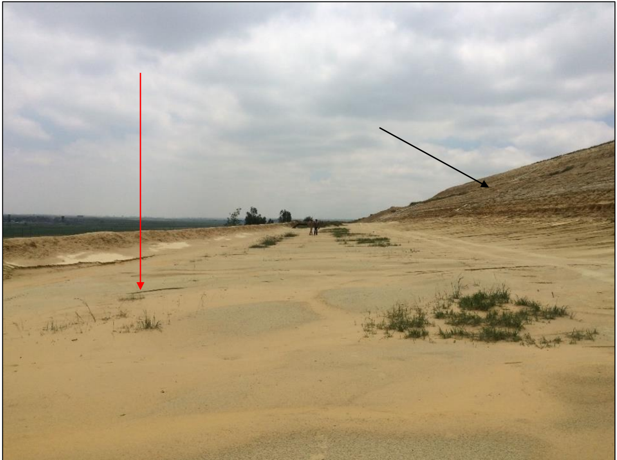
Figure 3.29: Buried trial plots on berm area of the Rooikraal TSF site next to eroded TSF slope (right) with Eragrostis curvula grass canopies projecting above the deposited mine tailings. E. curvula grass canopies are indicated by a red arrow and the eroded TSF slope is indicated by a black arrow. Photo taken by C.A. Kruger, 15/11/2016.
