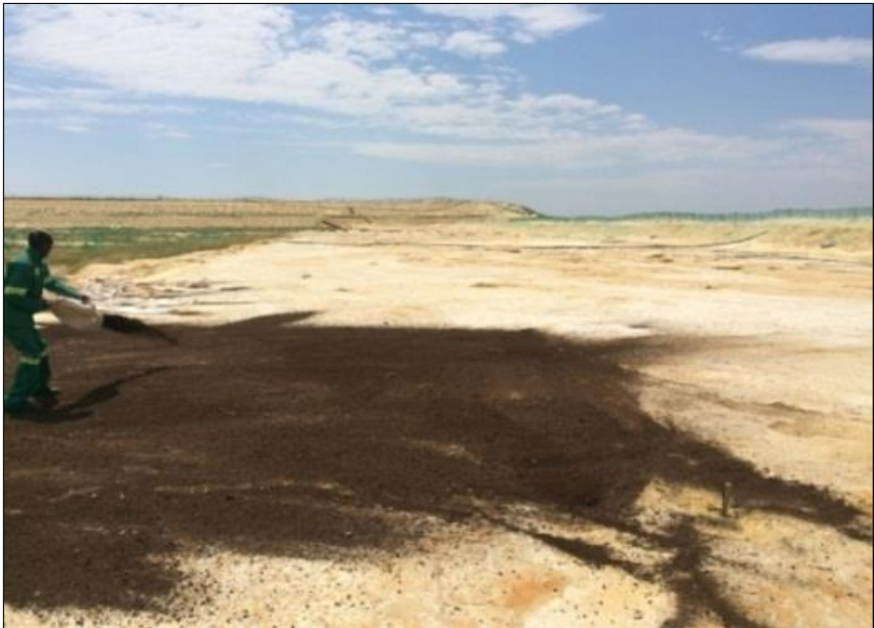
Figure 3.13: Dolomitic lime applied to the bare top-flat trial site on Crown gold TSF site to neutralise the tailings acidity. Photo taken by C.A. Kuger, 20/2/2016.
