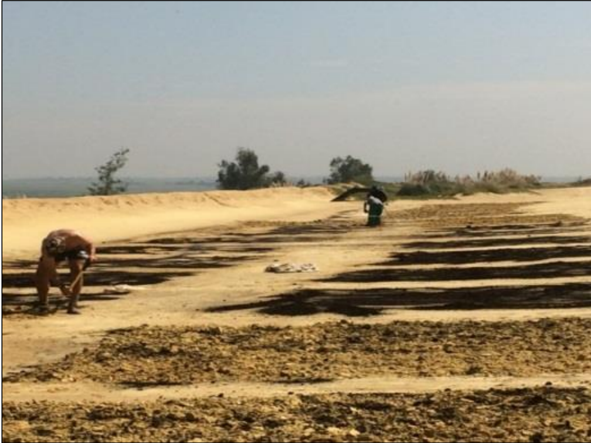
Figure 3.16: Lime and compost being worked into the tailings surface manually after application at the Rooikraal gold TSF site. Photo taken by C.A. Kruger, 24/2/2016.
