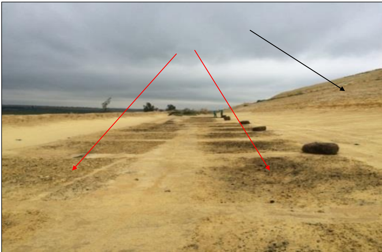
Figure 3.4: Ameliorated trial plots, indicated by red arrows, during mulching after seed treatments were sown at the Rooikraal gold TSF next to TSF slopes characterised by gully and rill erosion on the right. TSF slopes are indicated by a black arrow. Photo taken by C.A. Kruger, 9/3/2017.
