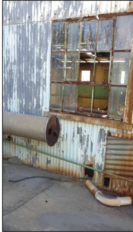
Figure 78: Pipe end that previously supplied air to workshops
