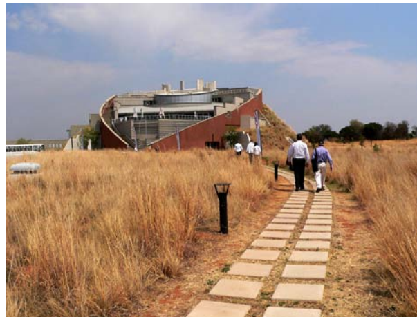
Figure 6.7: View from north of The Tumulus Building Exhibition Centre, Cradle of Humankind (COH)
