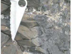
7 Dolerite dyke in cutting on Baobab Hill on the main road, south of Pafuri.
