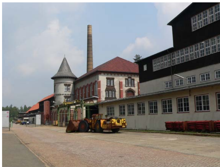
Figure 3.1: Part of the Rammelsberg reduction works, Rammelsberg World Heritage Site (WHS), Germany
