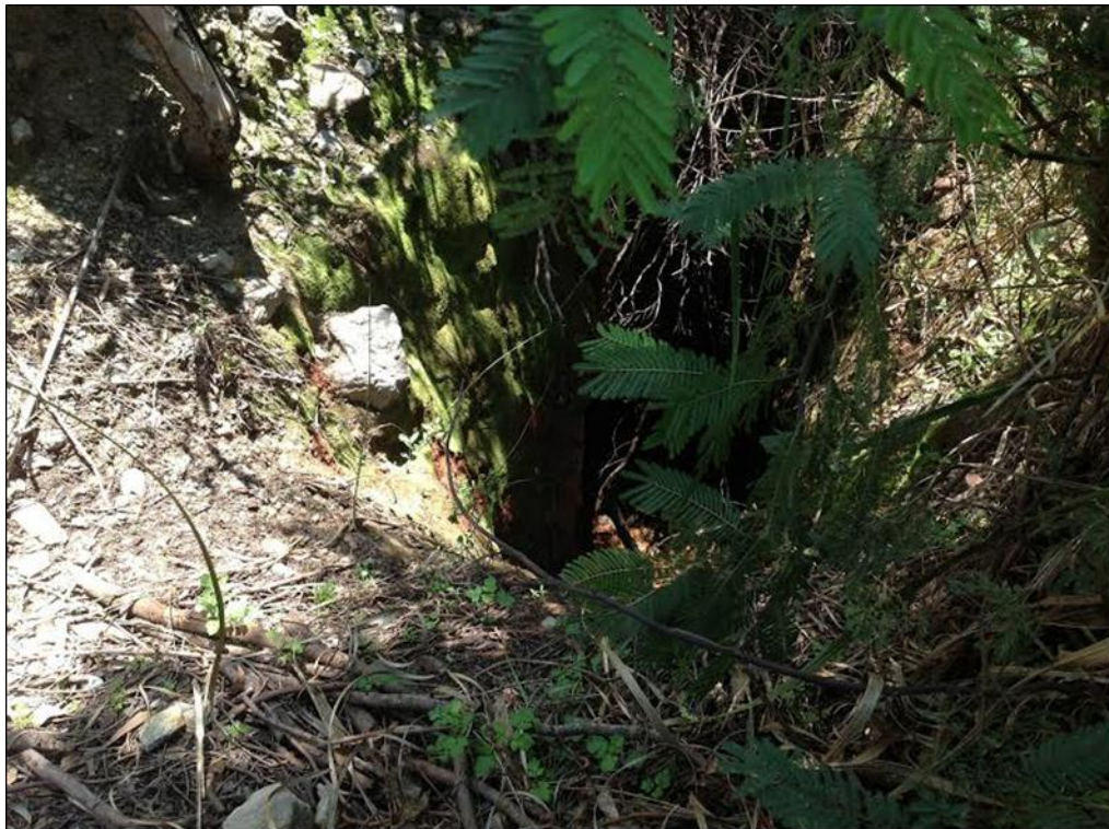
Photo 3.2: Adit allowing access to shallow underground workings
