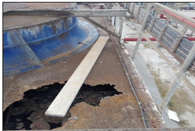
Figure 30: Mine A PCT damaged deck 19
