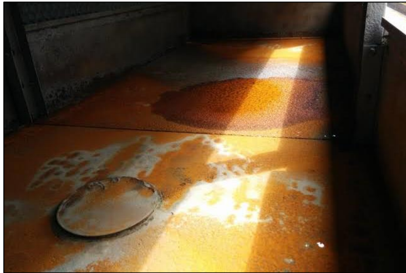
Figure 15: Corroded PCT 12
