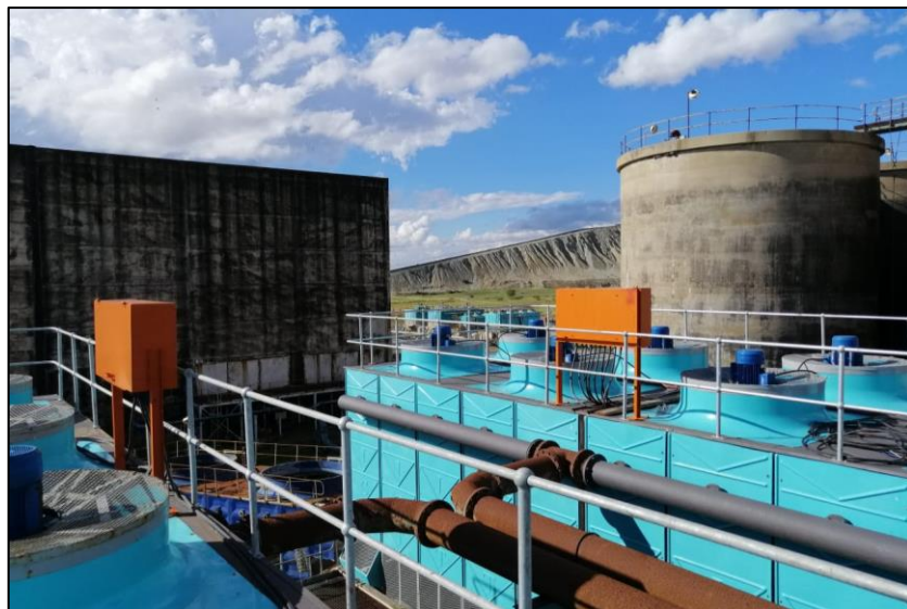
Figure 33: New galvanised pipeline installed 22
