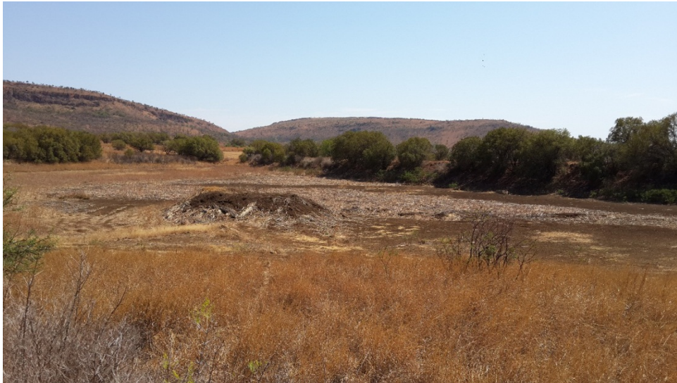
Figure 4.7: Sediment mound waiting to be taken away from a cleaned dam.
