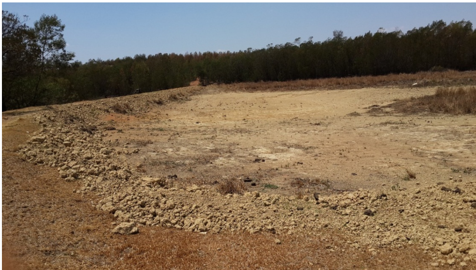
Figure 4.7: Sediment mound waiting to be taken away from a cleaned dam.
