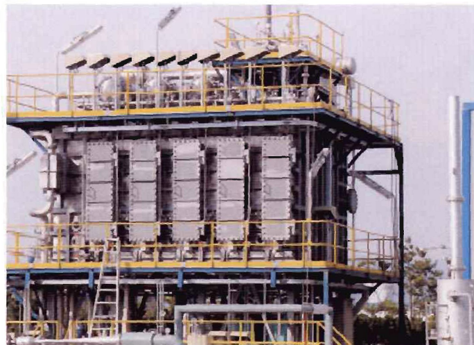
Figure 2-1: MED plant with horizontal tubes
