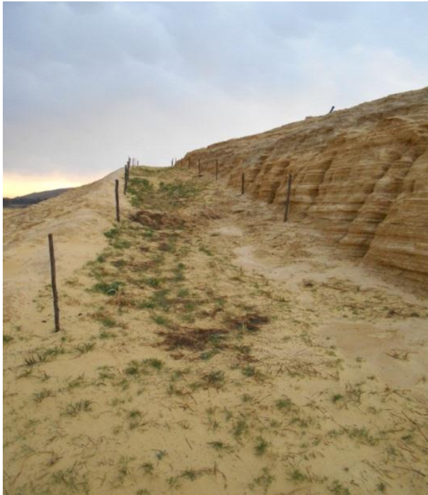
Figure 5.8: Rooikraal TSF second survey for growth and survival results (Photo: H Taute, August 2015); damage due to tailings spillage indicated by the arrow.
