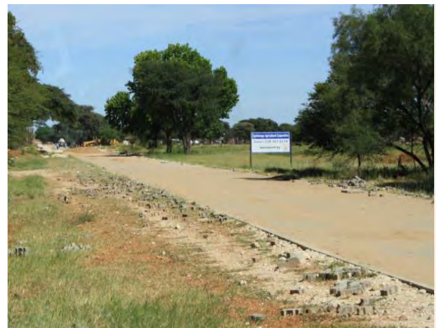
Figure 55: Upgrading of roads Source: Personal source (2013)
