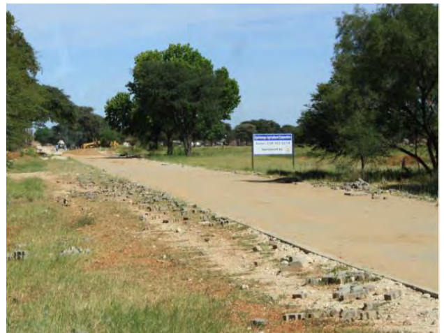
Figure 55: Upgrading of roads Source: Personal source (2013)
