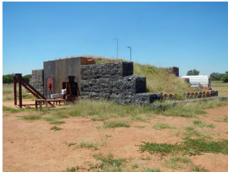
Figure 85: Paardefontein test range bunker
