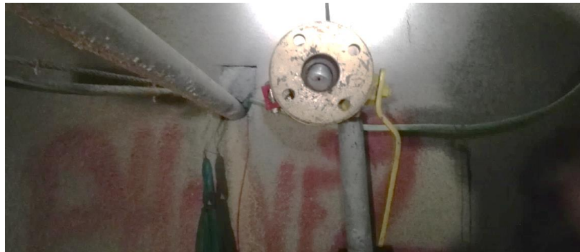
Figure 25: Installed new refuge chamber valve 28
