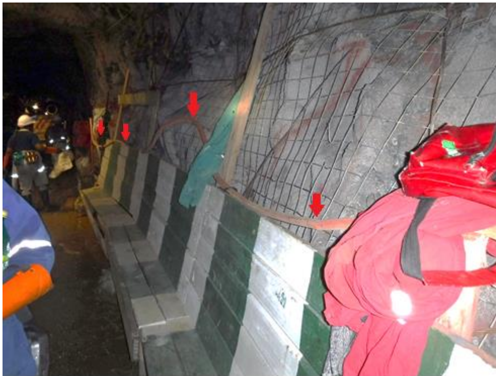
Figure 40: Compressed air being abused for cooling
