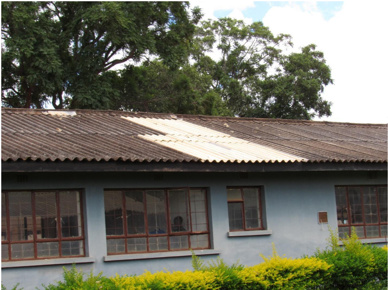
Figure 5-17: Replaced asbestos roof after an inferno in a laboratory at Chalimbana University (Source: Researcher's archive, 2022/2023)
