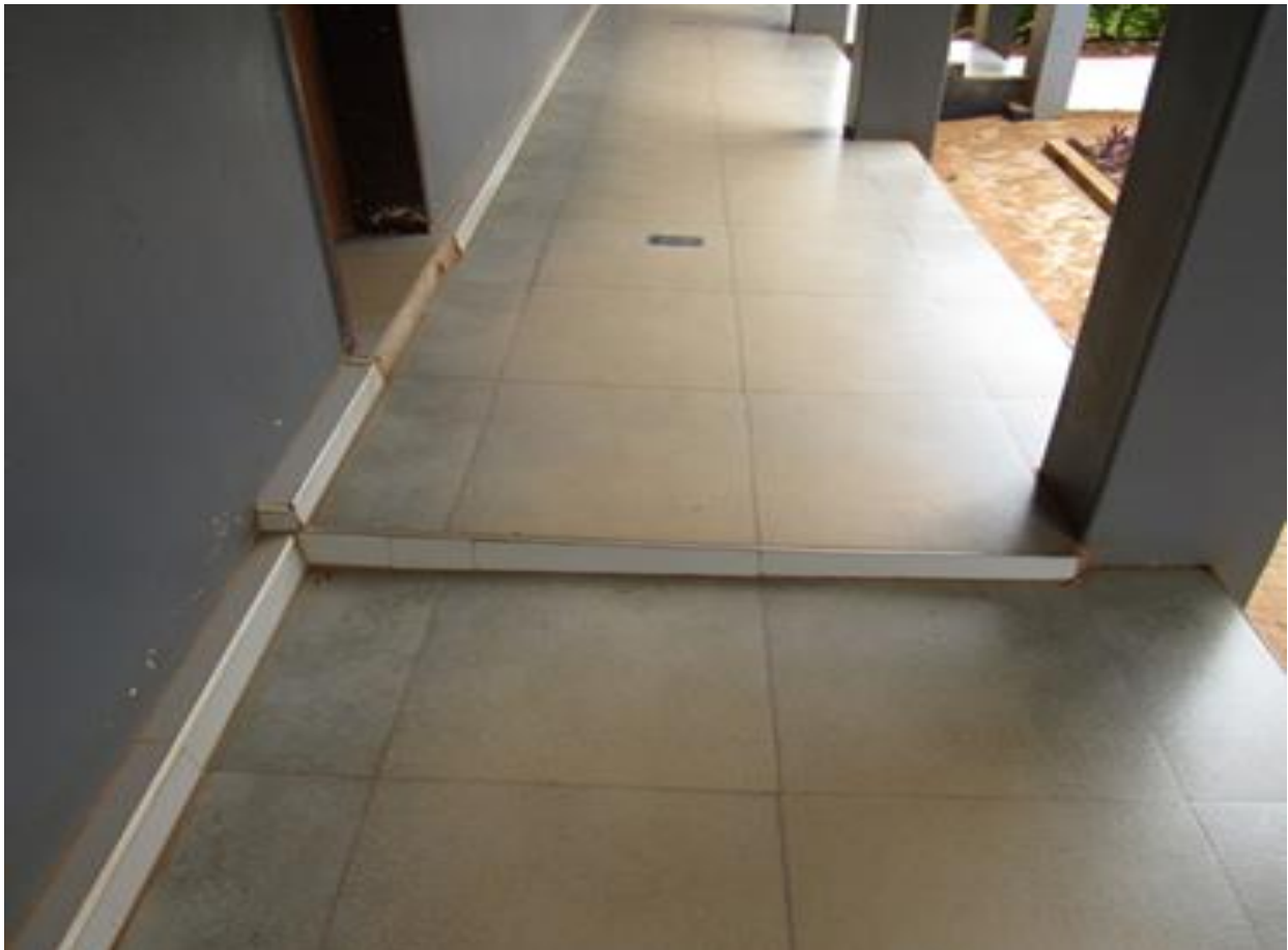
Figure 5-6: A step along a corridor at Chalimbana University (Source: Researcher's archive, 2022/2023)
