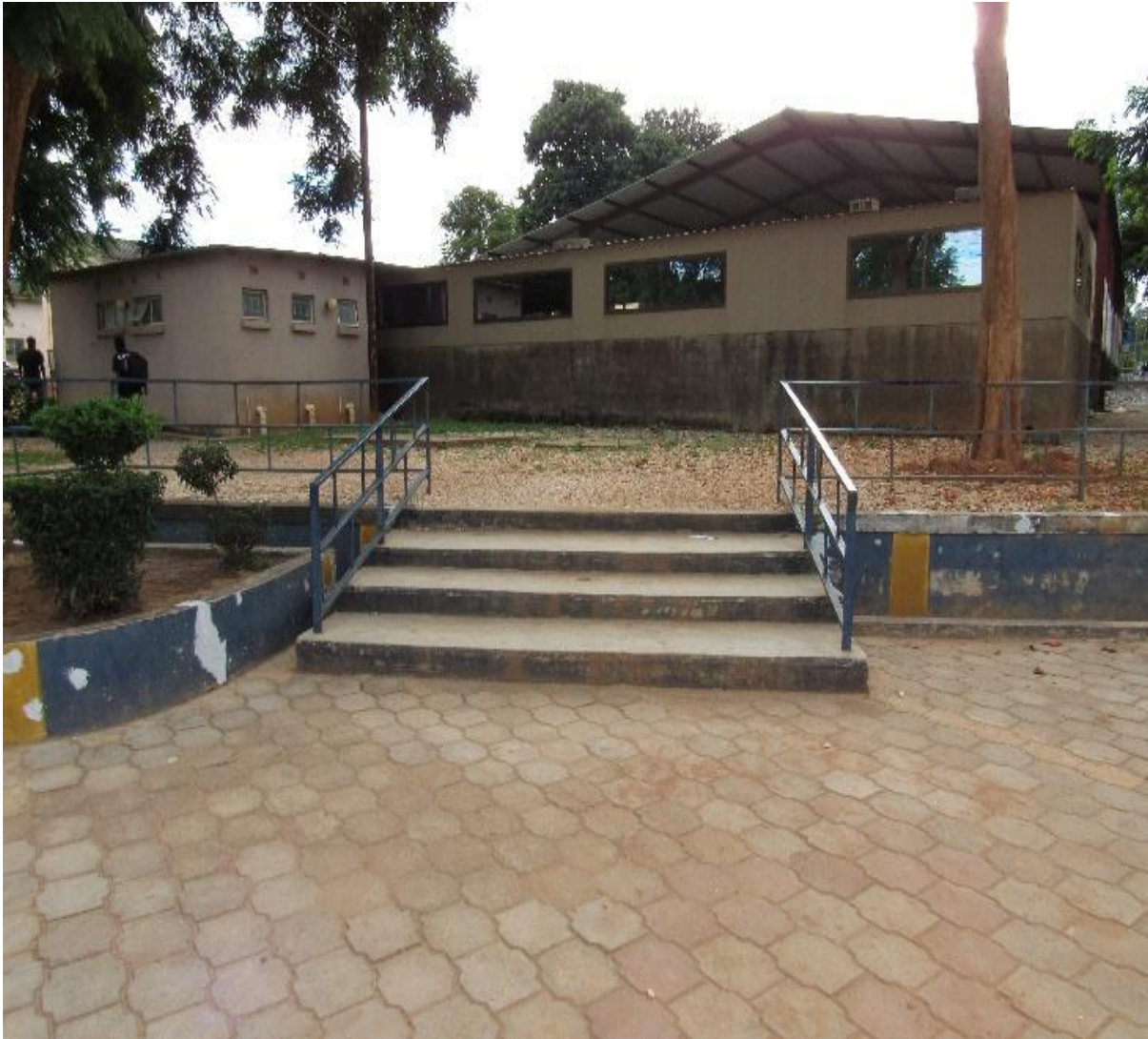
Figure 6-3: Staircase with guard rails at Chalimbana University (Source: Researcher's archive, 2022/2023)
