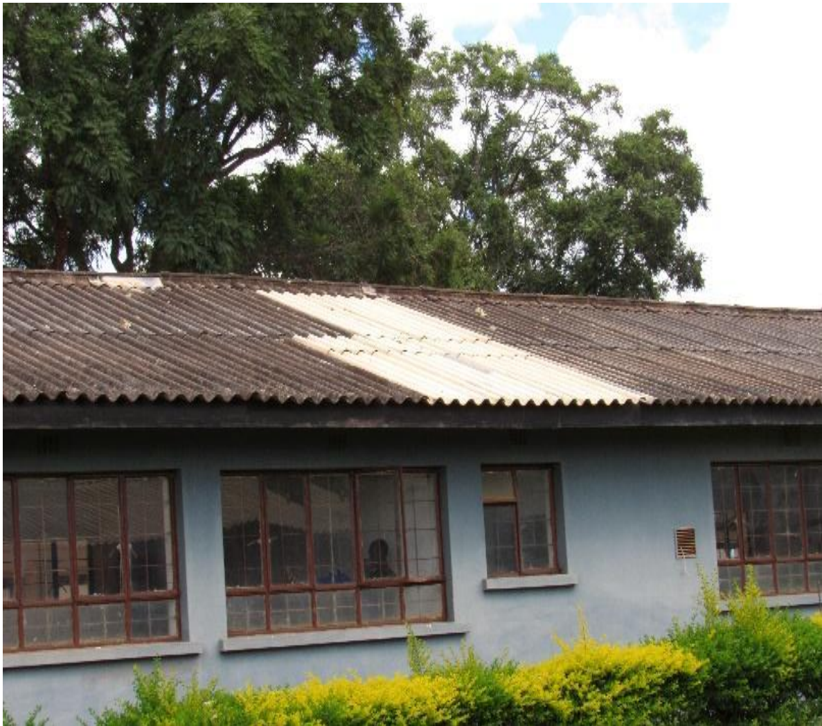
Figure 5-13: A building block with an asbestos rooftop at Chalimbana University (Source: Researcher's archive, 2022/2023)
