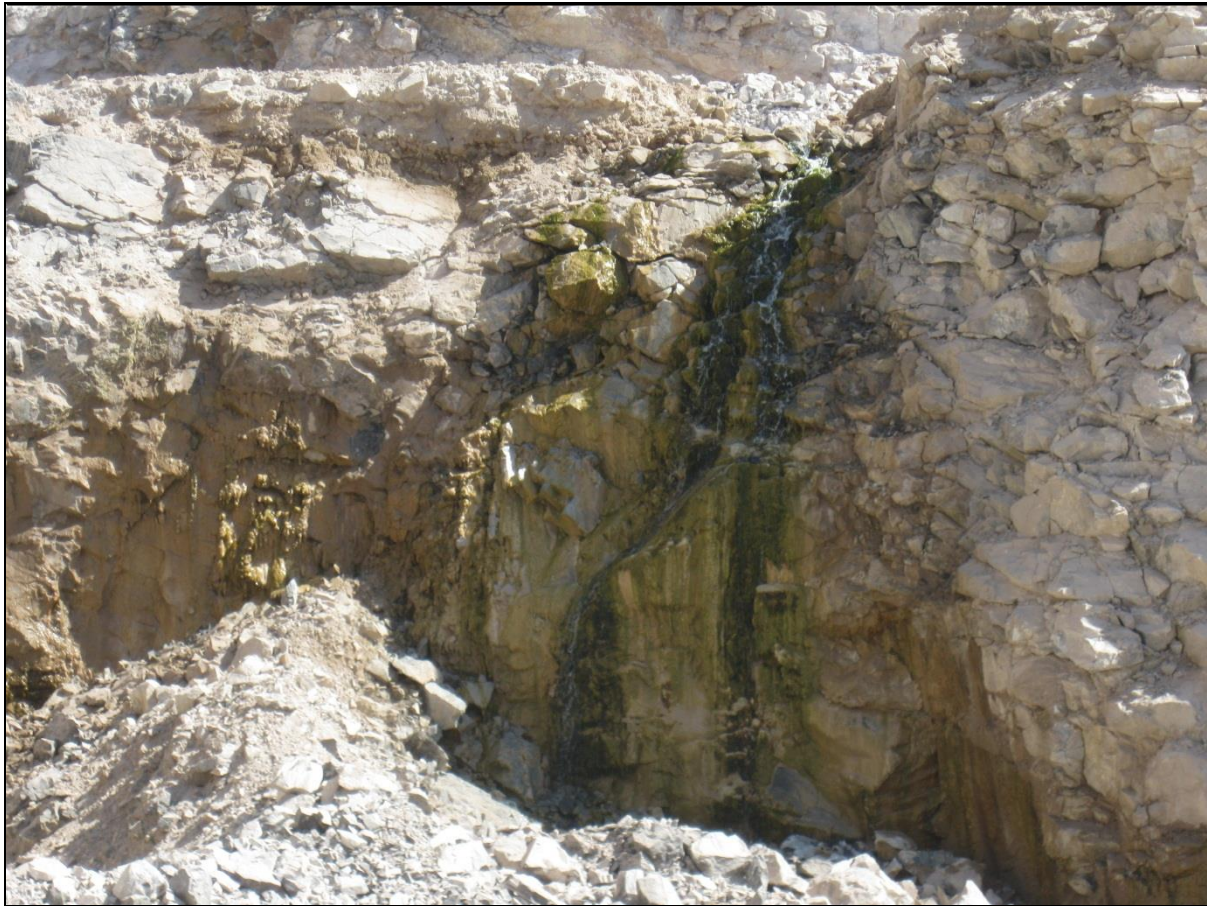
Figure 6.25: Fractured quarry wall with Cr(VI) polluted seepage
