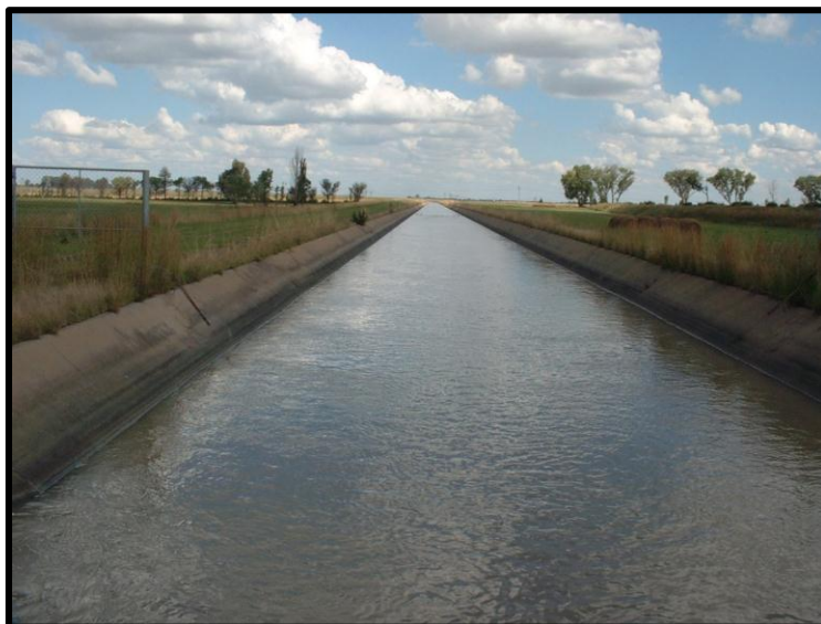
Figure 3.2 Twenty kilometre long canal (with a hydraulic retention time of 4 – 6 hours), supplying source water to the Zuikerbosch DWTW.
