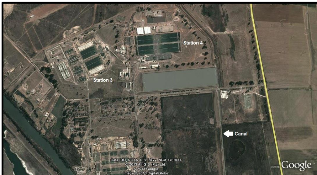
Figure 3.3 Google Earth picture of stations 3 and 4 at the Zuikerbosch DWTW (Google Earth, 2013).
