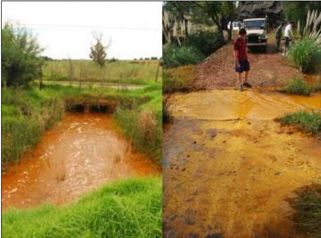
Figure 2.4: Right: The AMD contaminated Tweelopiespruit flowing under the R24 road into the Krugersdorp game reserve. Left: Water flowing out of the game reserve's aviary dam showing clear signs of contamination (Earthlife Africa, 2015).
