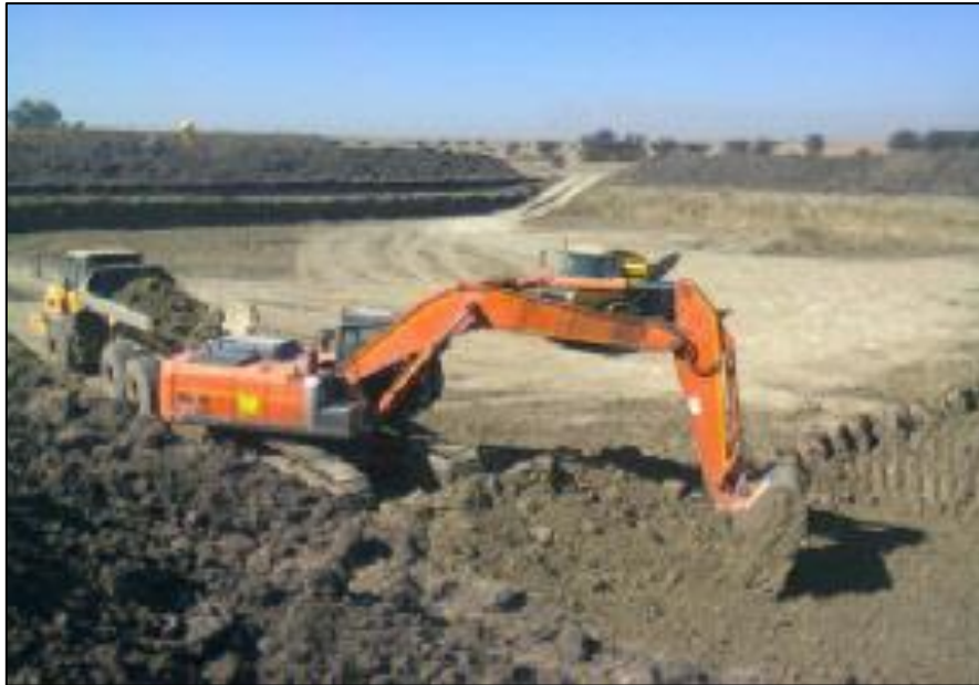
Figure 2.20: Bentonite excavation at Yellowstar bentonite quarry (Yellowstar Bentonite, 2015)
