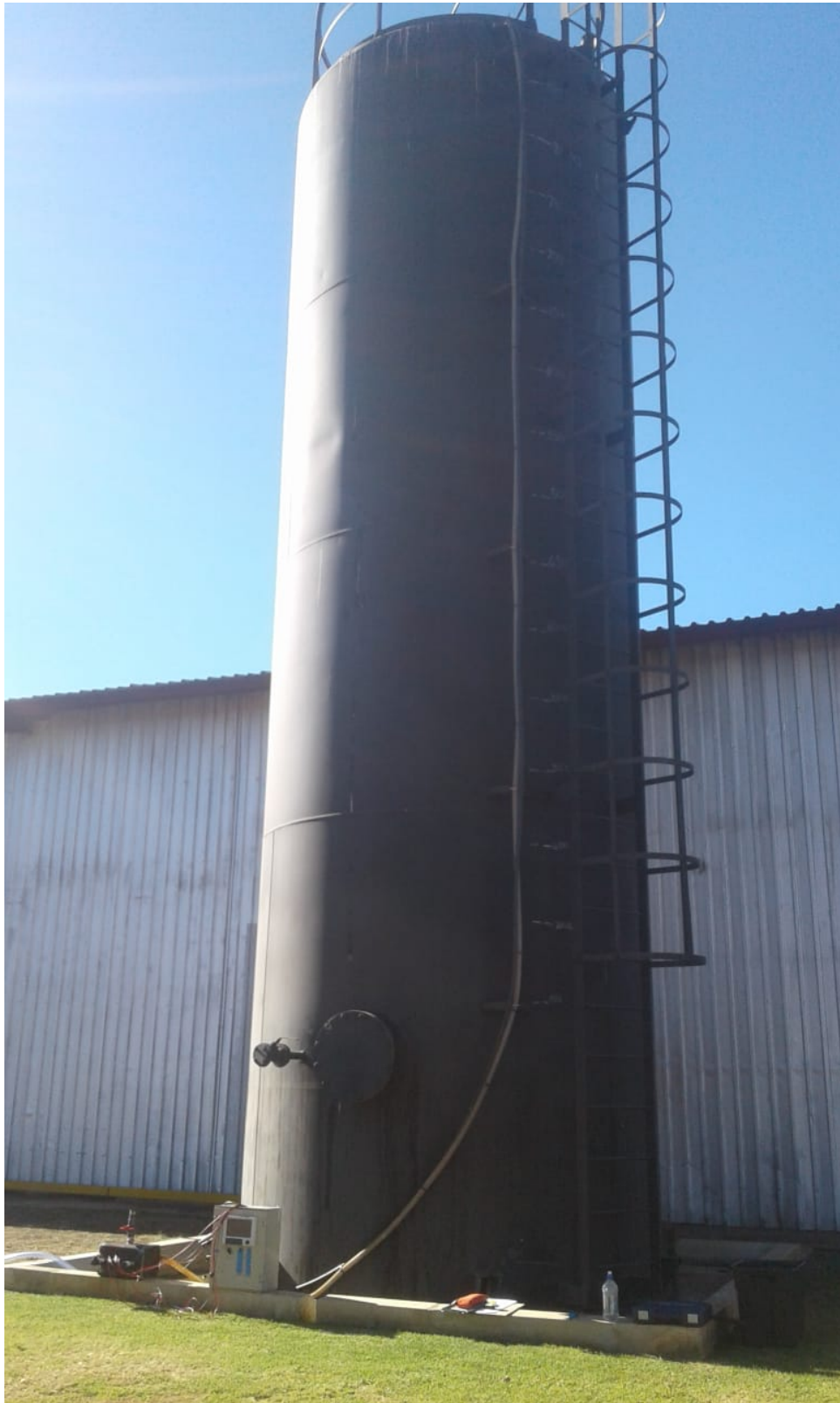
Figure 4.32. WJ Engineering Hydro Test Facility large water tank
