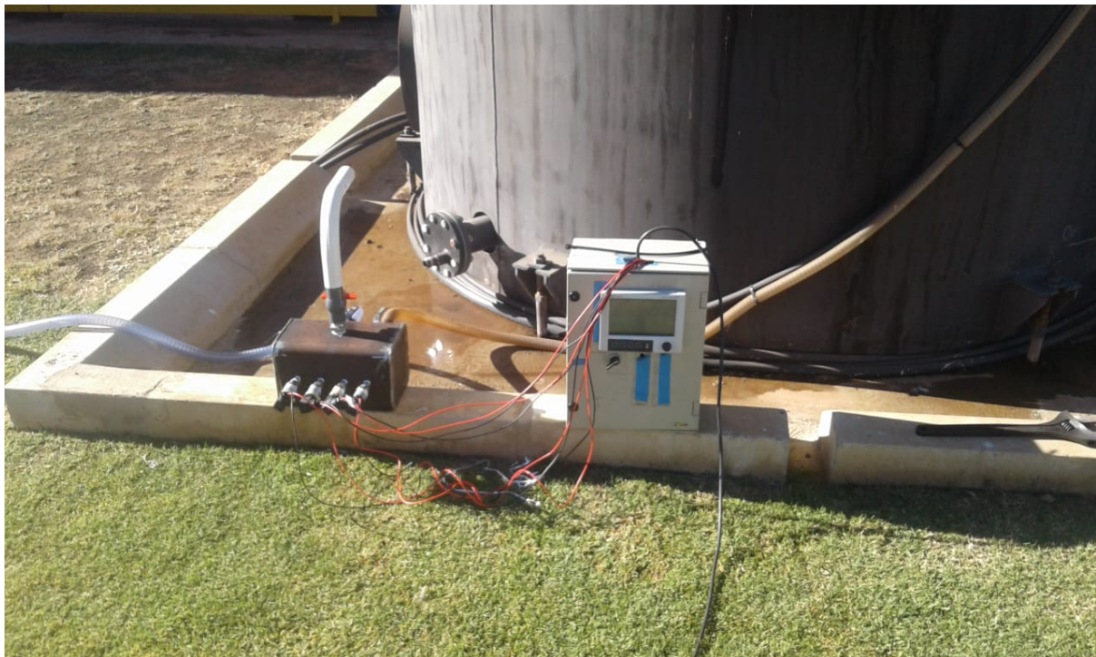
Figure 4.31. Pressure sensors installed for calibration
