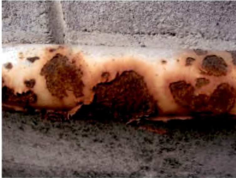
FIGURE 130: CORRODED PIPE
