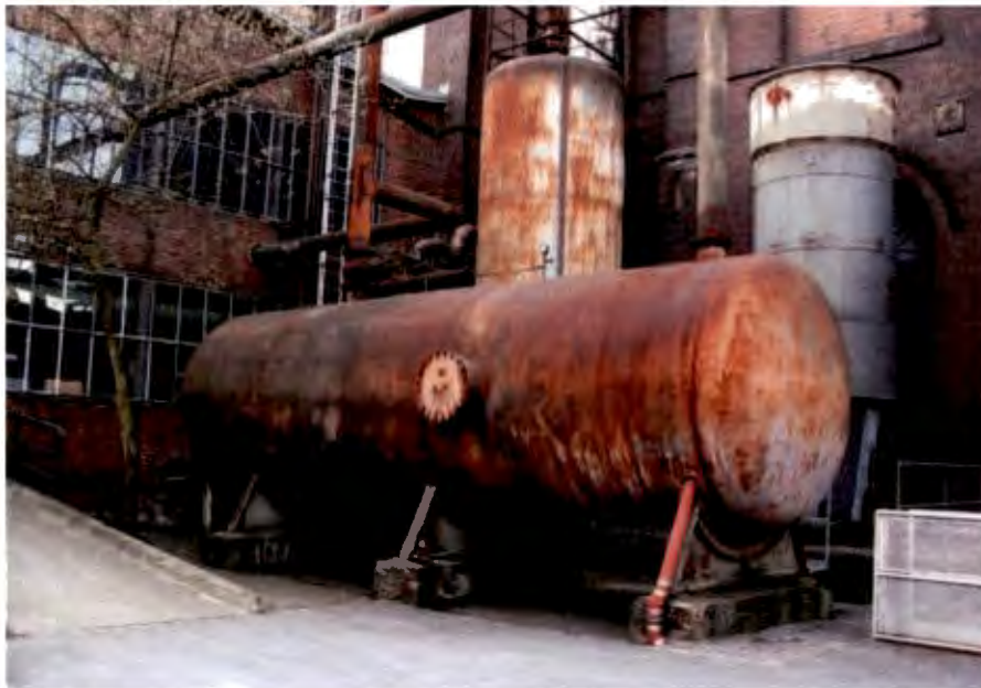
FIGURE 131: CORRODED PRESSURE VESSEL
