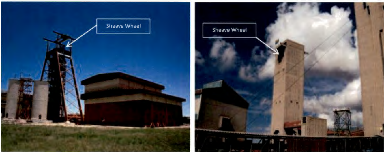
FIGURE 1: SHEAVE WHEELS IN HEADGEARS IN UNDERGROUND MINES.
