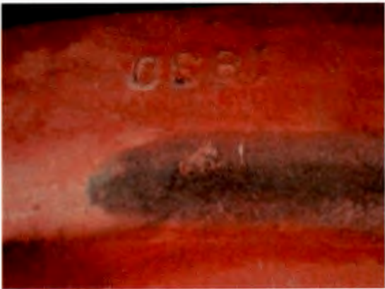
FIGURE 10: WEB WEAR LIKELY DUE TO AN INCORRECT FLARE ANGLE
