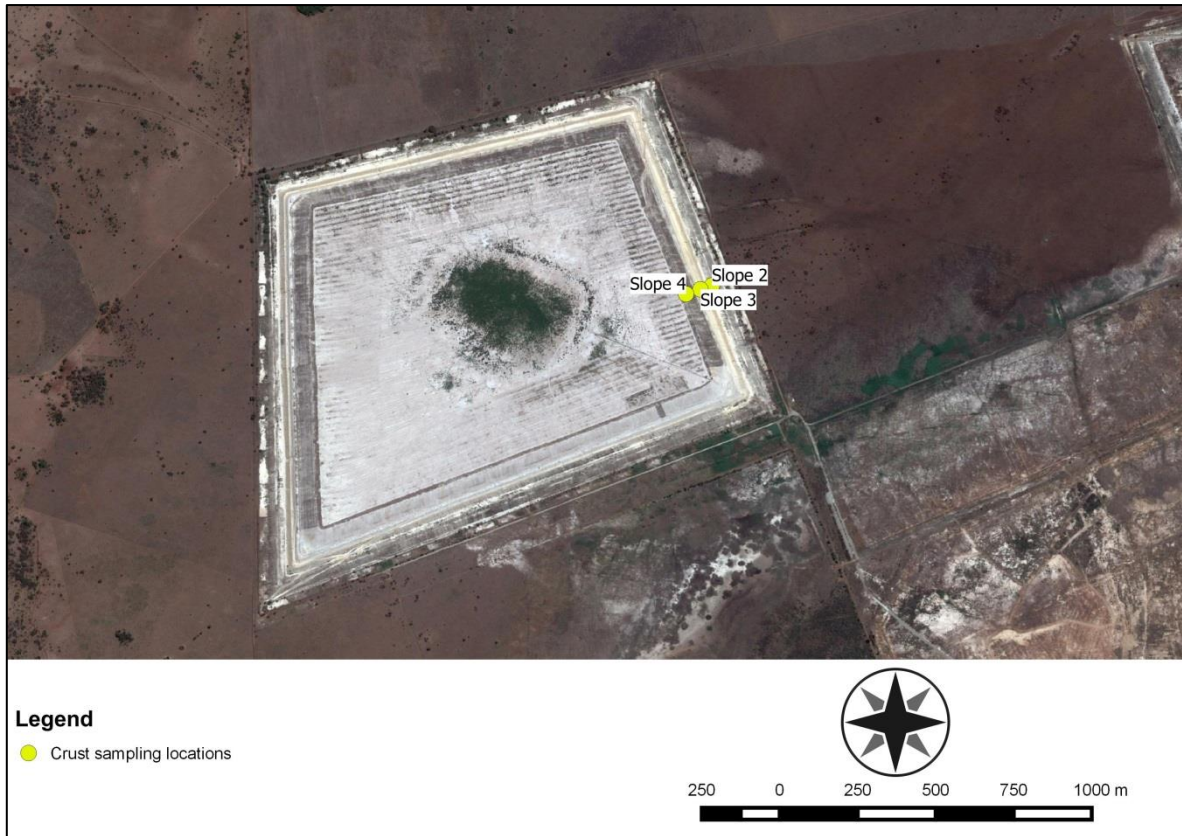
Figure 15: Locations of composite tailings sampling in the Chemwest 5 TSF.
