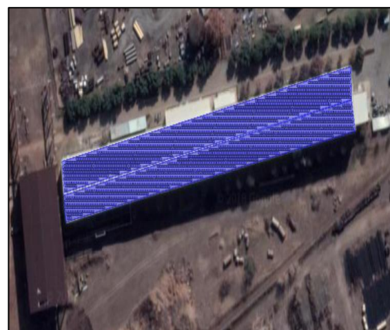
Emhlangeni Workshop 618.6 kWp
