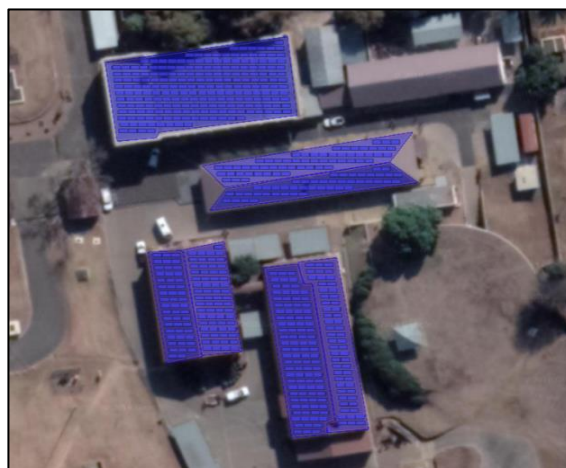
Zwartkopjes Administration 188.5 kWp
