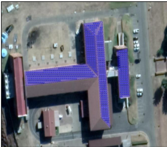
Zuikerbosch Administration 157.4 kWp
