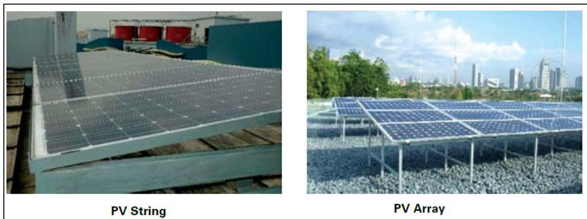
Figure 10: PV string and PV array [37]
