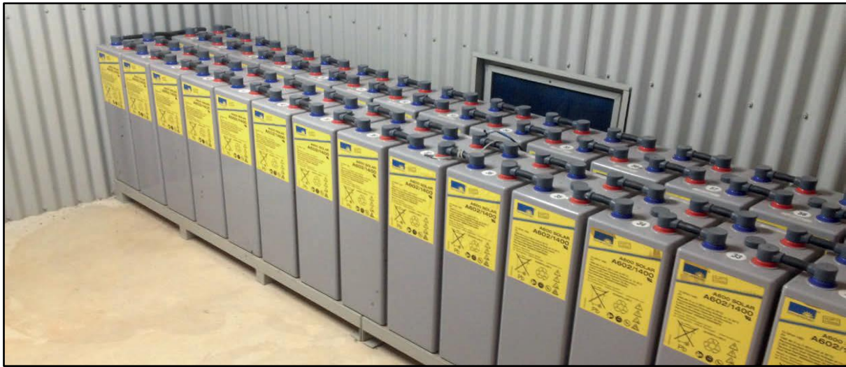
Figure 12 Battery bank [44].
