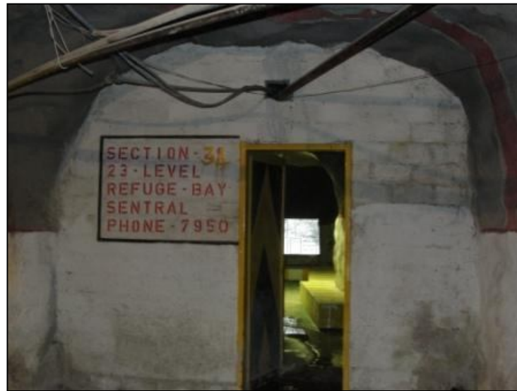
Figure 15: Underground refuge bay [37]
