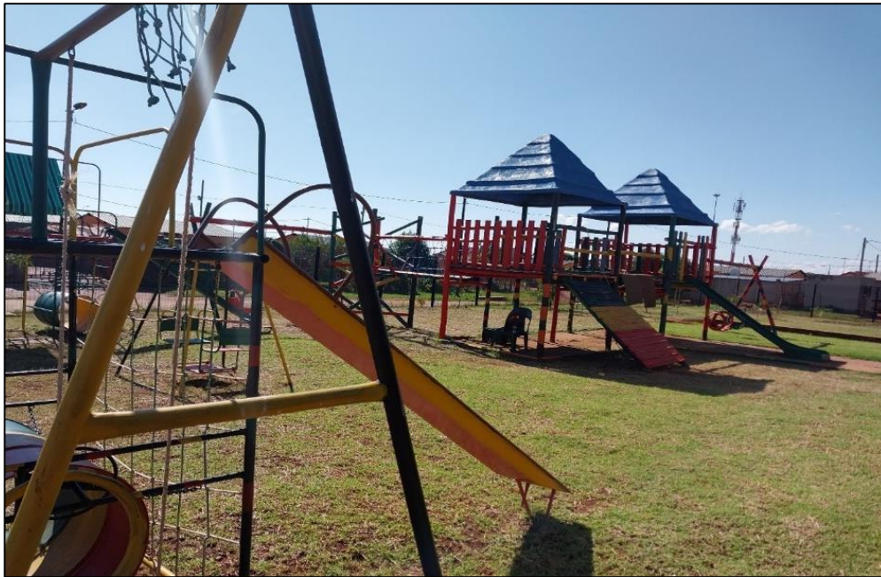
Figure 4.9: ECD centre's play facilities and adjacent low-cost houses
