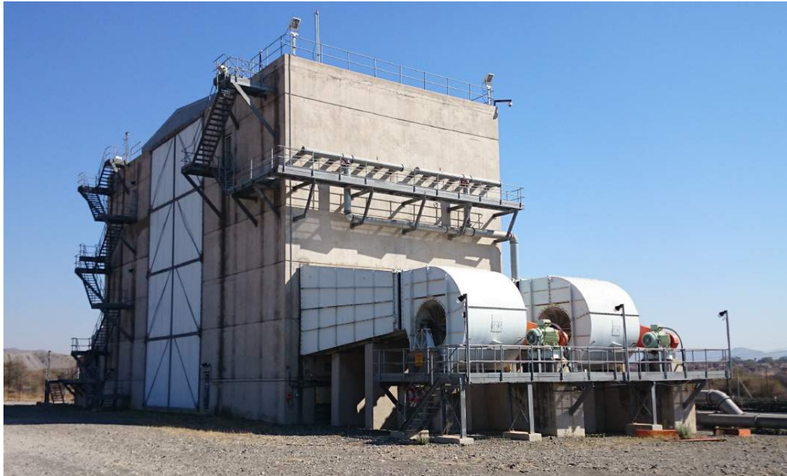
Figure 3.2: BAC on site
