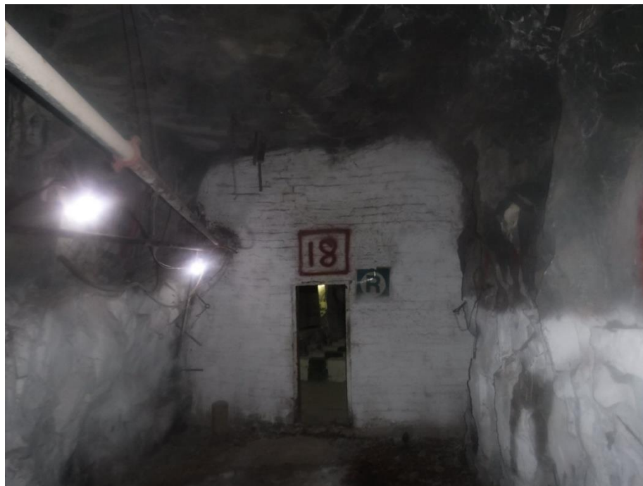
Figure 16 - Typical refuge bay found in deep-level mines 2
