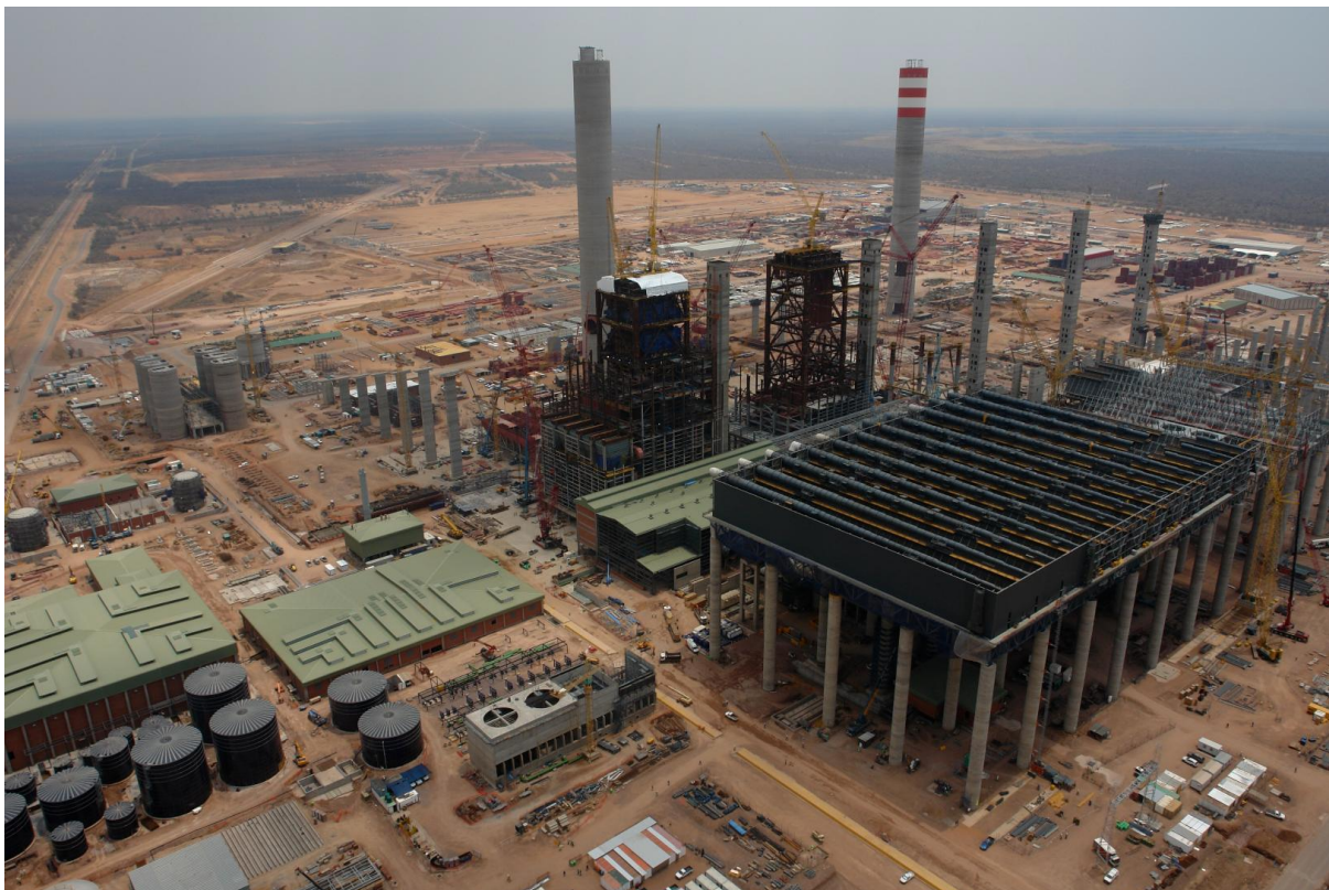
FIGURE 2-2: MEDUPI POWER STATION IN THE LEPHALALE AREA
