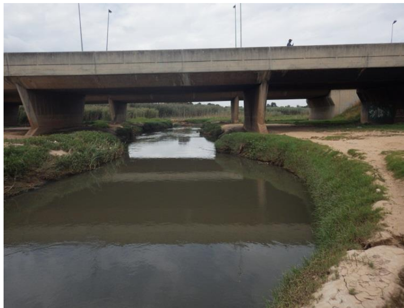
Figure 1.9: Sediment sampling site at Moroka located under the Chris Hani Road bridge
