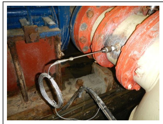
Figure B-12: Suction temperature probe
