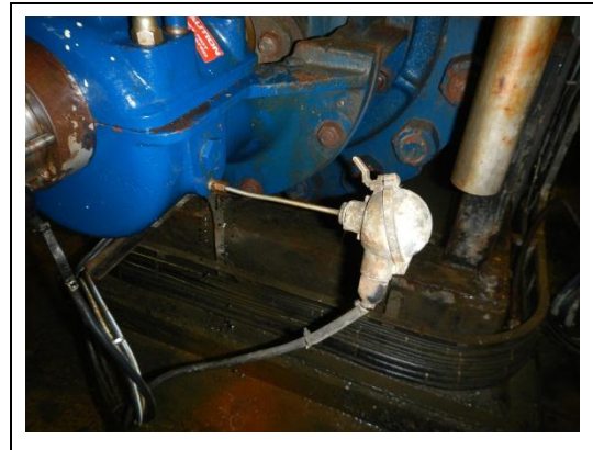
Figure B-22: Pump NDE temperature probe
