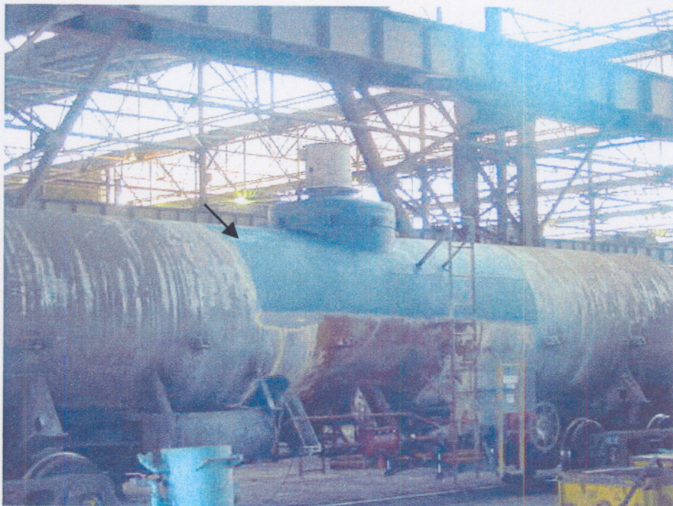
Figure 3.8: A view of the workspace (grey area) for the dome area work process
