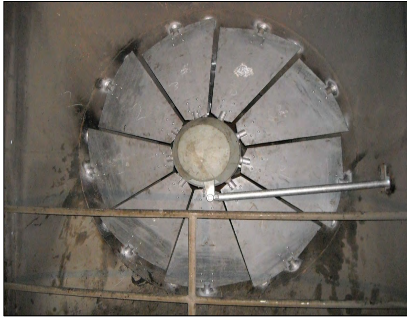
Figure 29: New improved IGV's.
