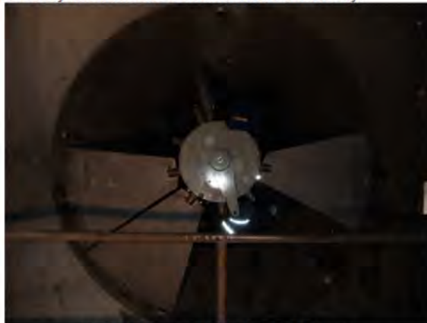
Figure 1: Alignment of the hub and the vanes
