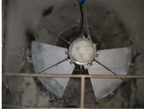
Figure 3: Alignment of the vanes
