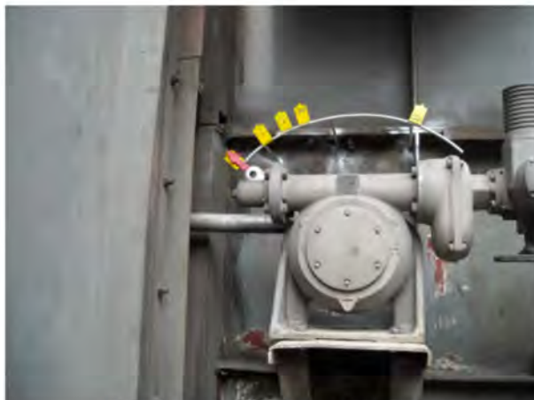
Figure 5: Angle indicators on the actuator
