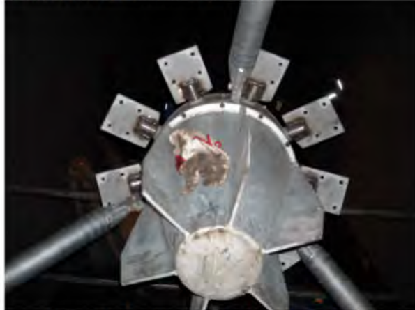
Figure 4: Vortex breaker bolted onto back of the hub
