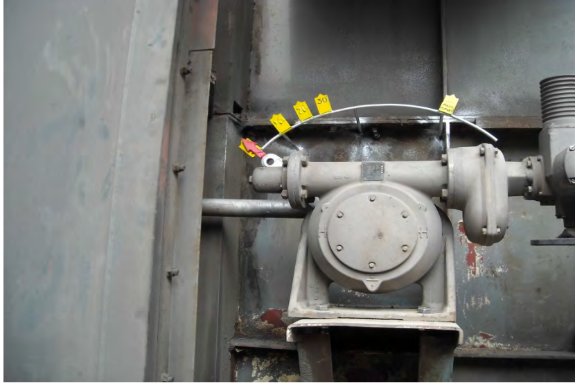
Figure 31: Electric actuator with angle indicators.
