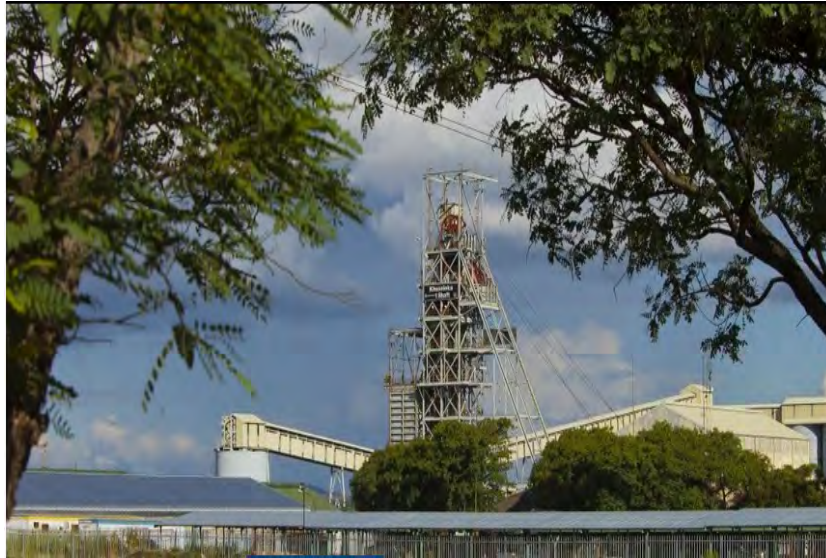
Figure 21: Mine A shaft [50].
