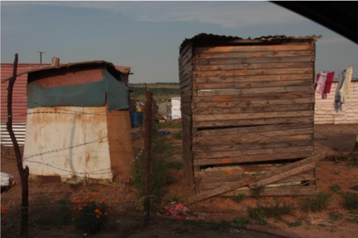
Illustration 4: On-site pit latrines constructed with salvaged material. (Photograph: JWN Tempelhoff).
