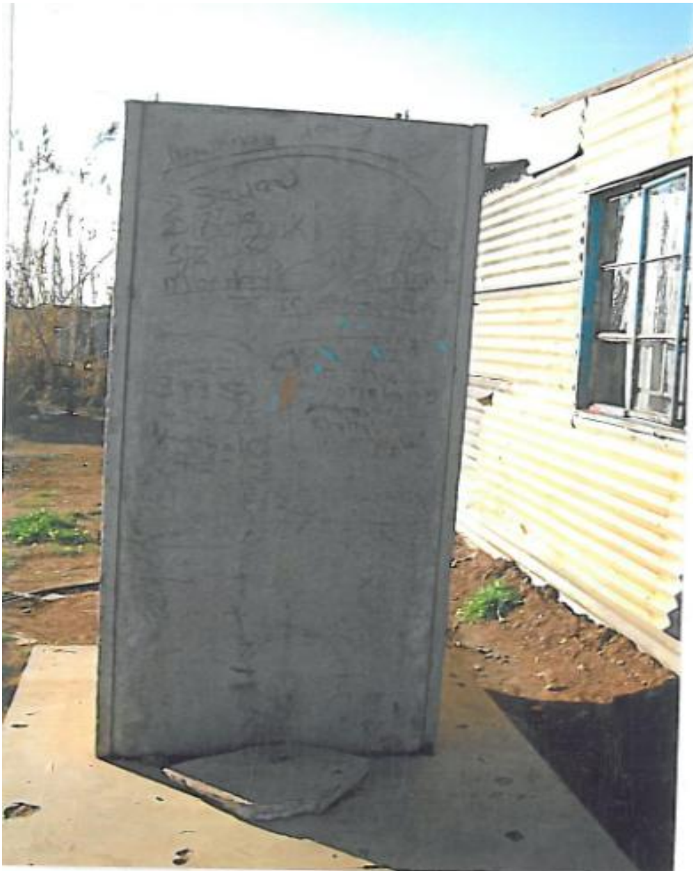
Illustration 8: Example of a slab toilet that local residents rejected in 1999. (Photograph: CT Musa).
