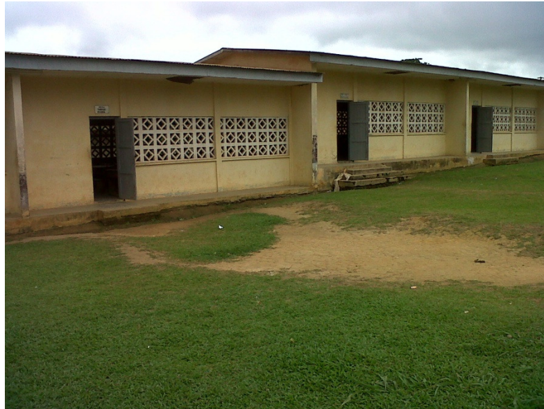
Figure 4.3: School from Remote Area
