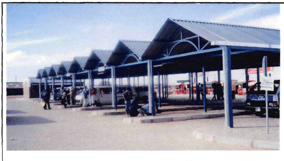
Photo 6: Complete taxi rank at Kalkspruit
