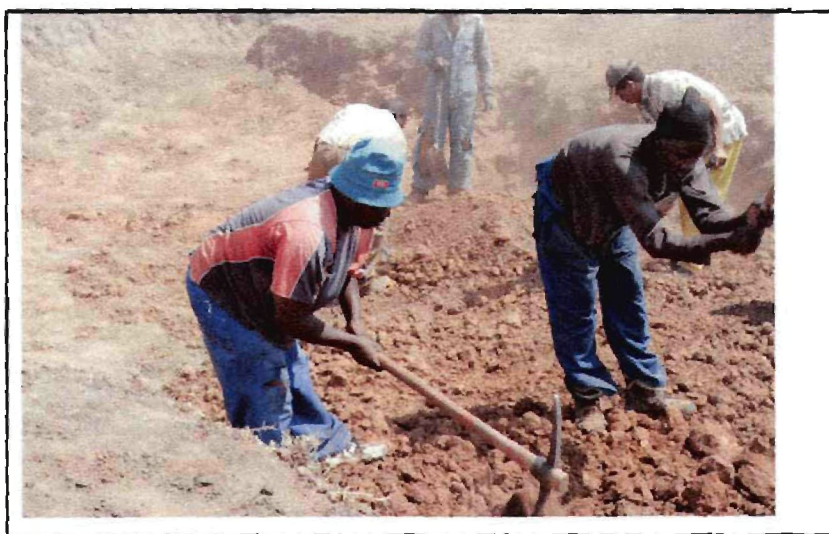
Photo 7: EPWP road construction at Ceres
