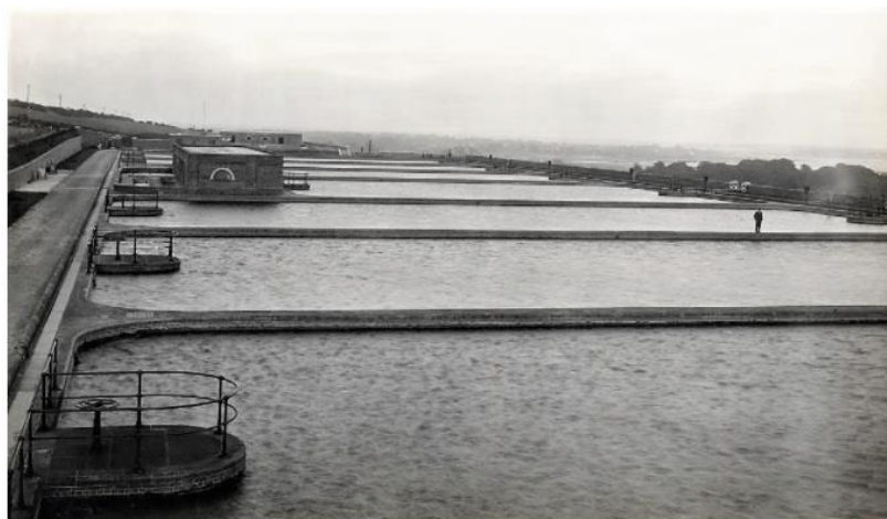
Figure 11: Large-scale slow sand filtration operation (Bruni & Spuhler, 2020).
