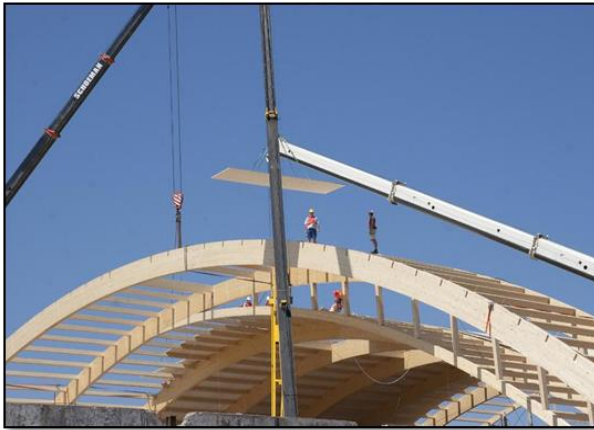
Laying of the roof
