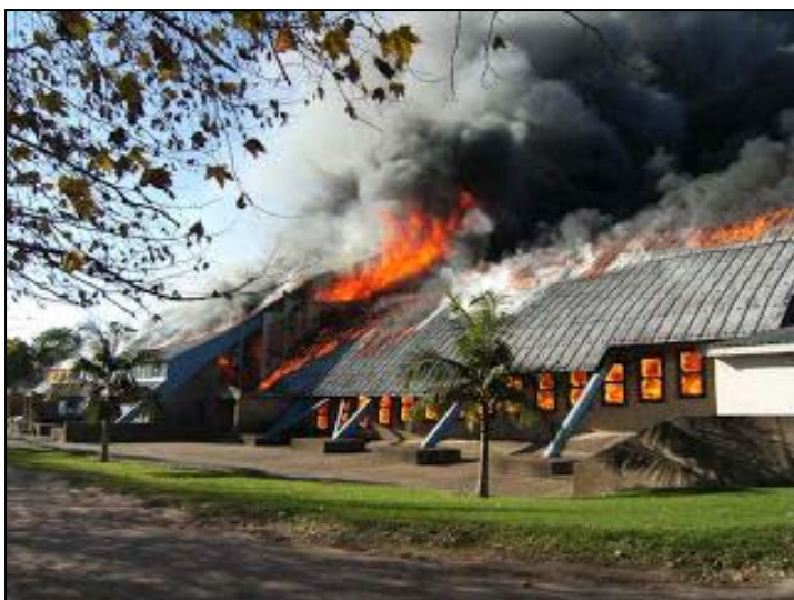
Figure 4.25: Auditorium destroyed by fire, 14 June 2008
