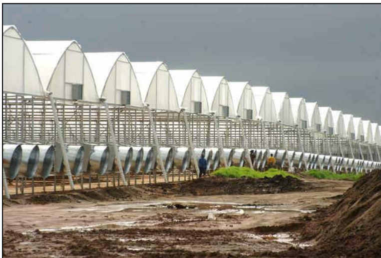
Figure 4.11: Construction of the hydroponic hothouses
