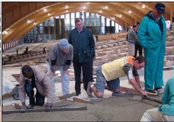
Leveling the auditorium floor
