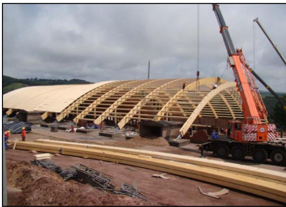
Erection of beams
