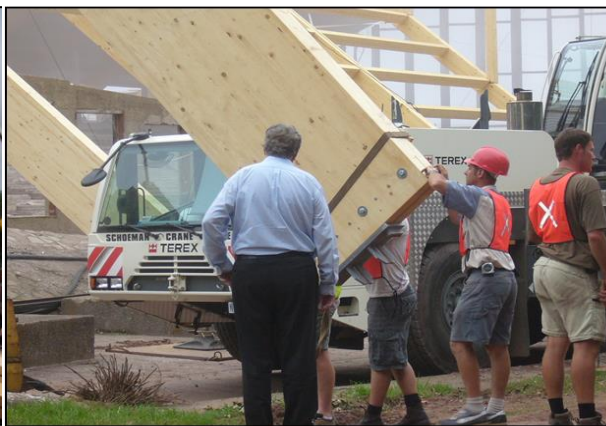
Fitting of beams of laminated wood from Europe
