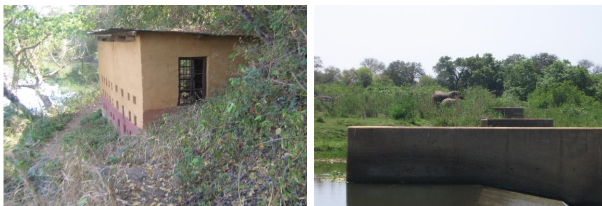
Figure 6-3: a) Pump station next to a holding dam which is the home of a hippopotamus, b) Elephant spotted close to a river irrigation pump station.
