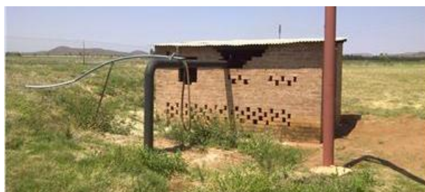
Figure 4: Pump station E36
