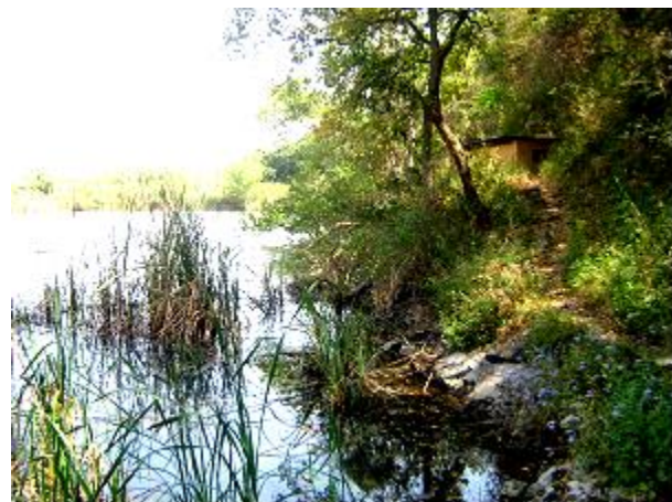
Figure 2: Pump station next to a holding dam housing a hippopotamus
