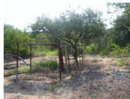
Figure 4: Pump station in the open veldt
