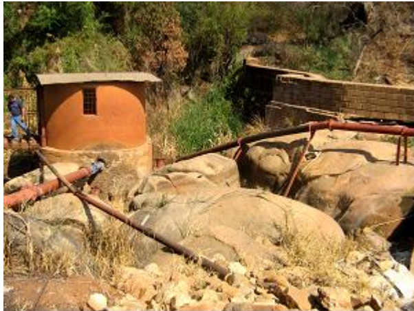
Figure 3: Pump station at the river
