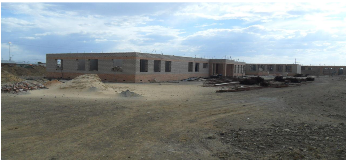
Figure 3.10: School D under construction
