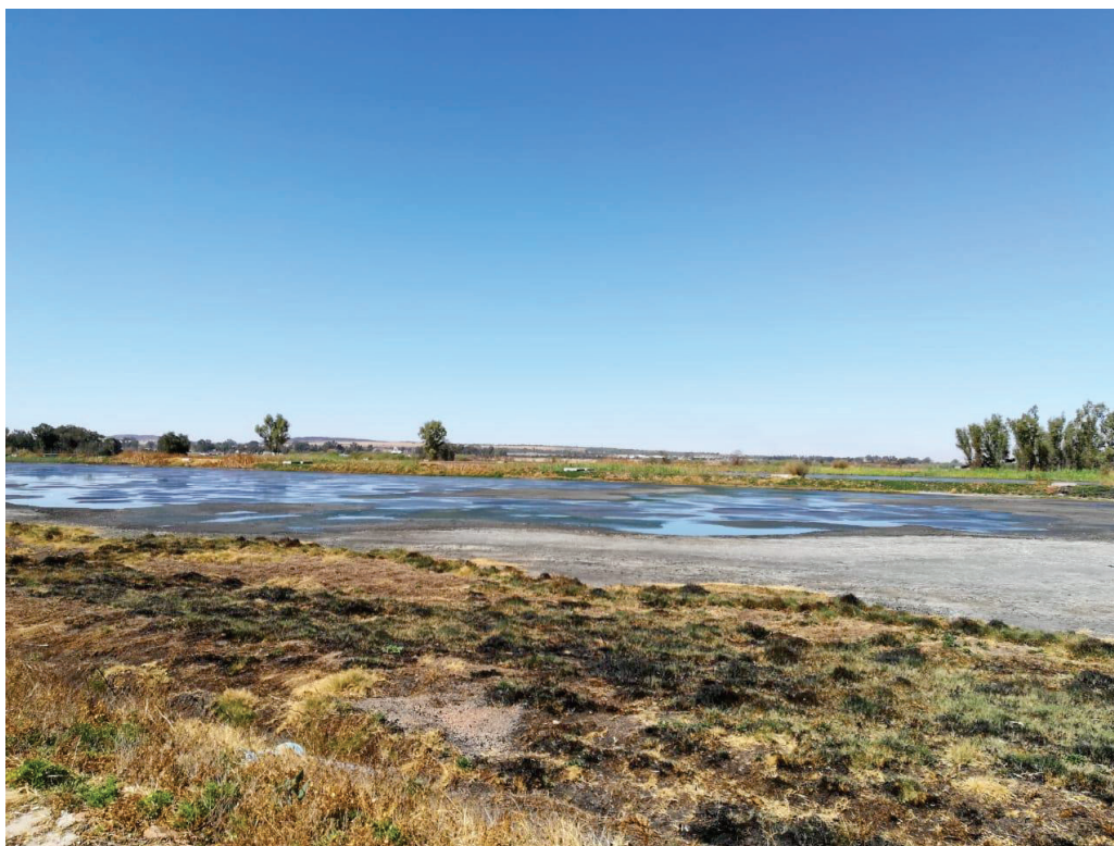
Figure 3-4: Municipal Discharged Sewage Sludge (DSS) dam.
