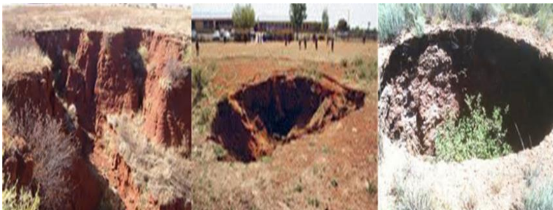
Figure 3.4 Sinkhole formations around mining around West Rand District Gauteng. Source: (Louw, 2011).
