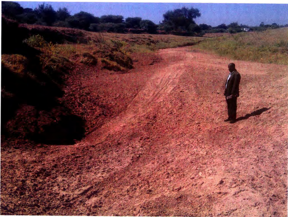
(a) A member of the Village Development Committee inspecting a river bed pit caused by sand mining
