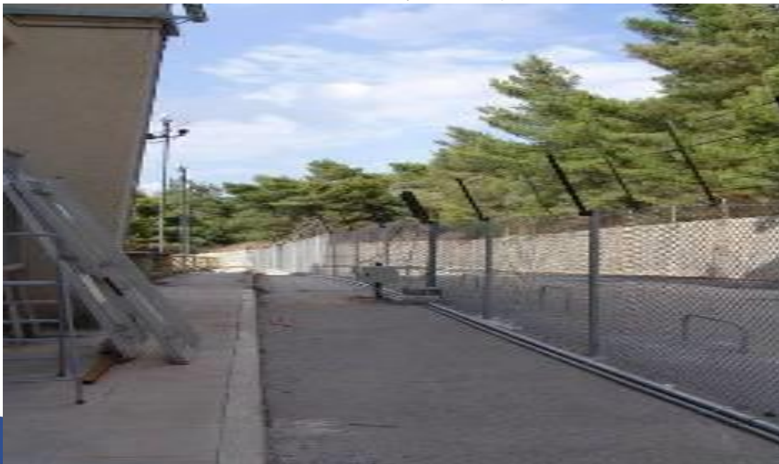
Figure 8: Double fencing and surveillance cameras – Physical Protection/Nuclear Security measures
