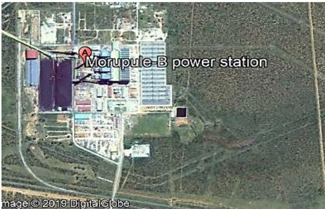
Fig. 3 - 2: Aerial view of Morupule-B Coal Thermal Power Station [ http://www.earth.google.com , Accessed April 26, 2019]
