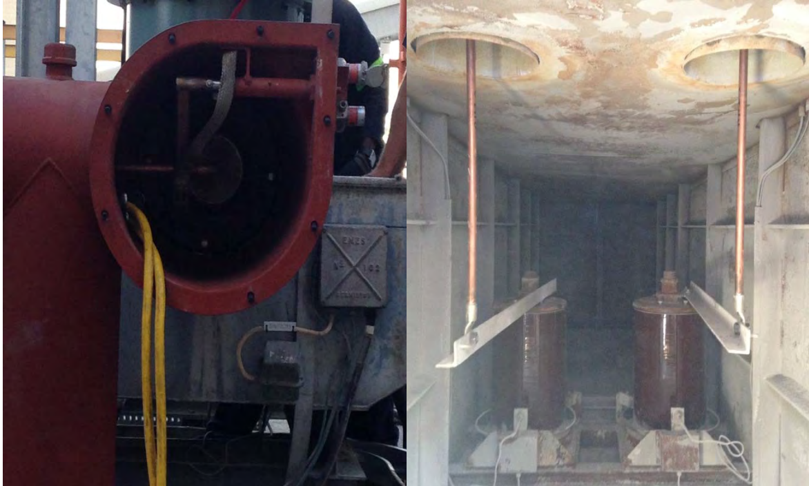
Figure 8-7: HV ducting modification into the ESP electrodes
