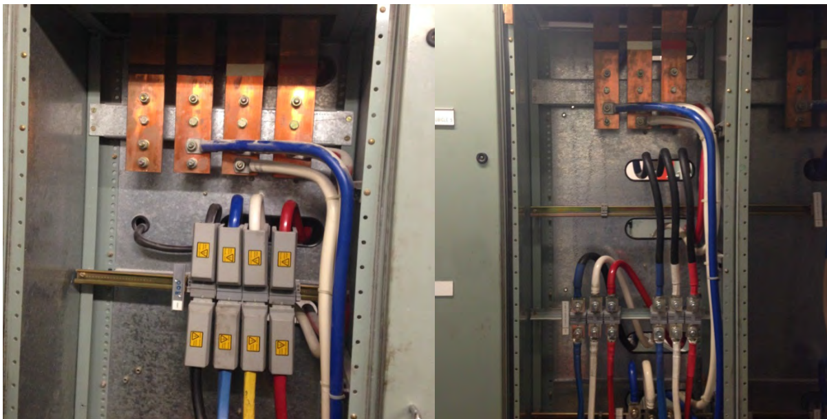
Figure 8-4: 380 V-board modification from 2-phase to 3-phase
