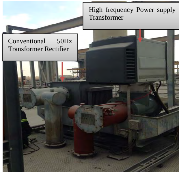
Figure 5: HFPS transformer installation
