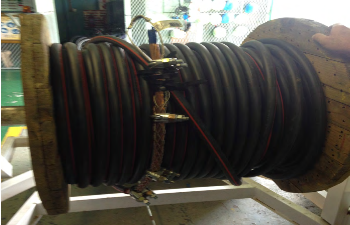
Figure 8-11: Sock method utilised for pulling the new 3-core cable onto the roof of the ESP
