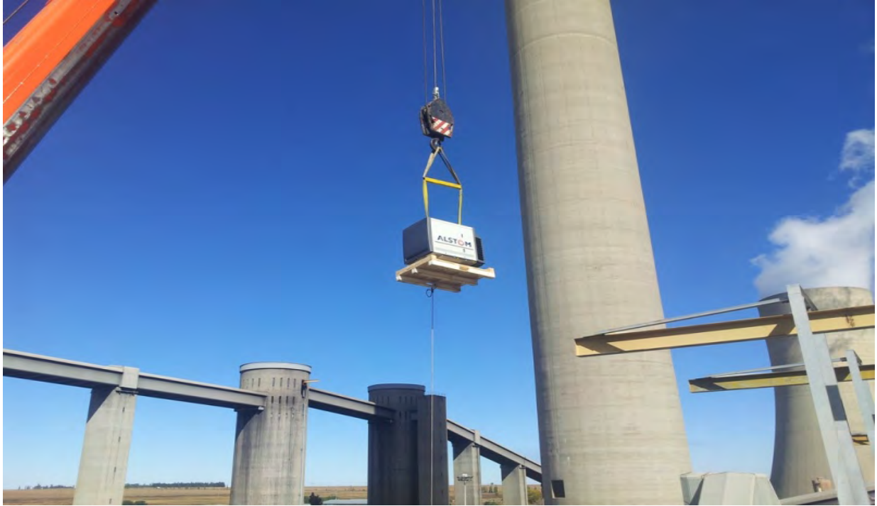
Figure 8-9: Hoisting of an HFPS onto the ESP roof for installation
