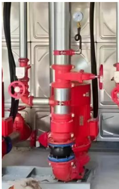
Figure 1-2: In-line rubber bellow application example (ChangYuanFlex, n.d.)
