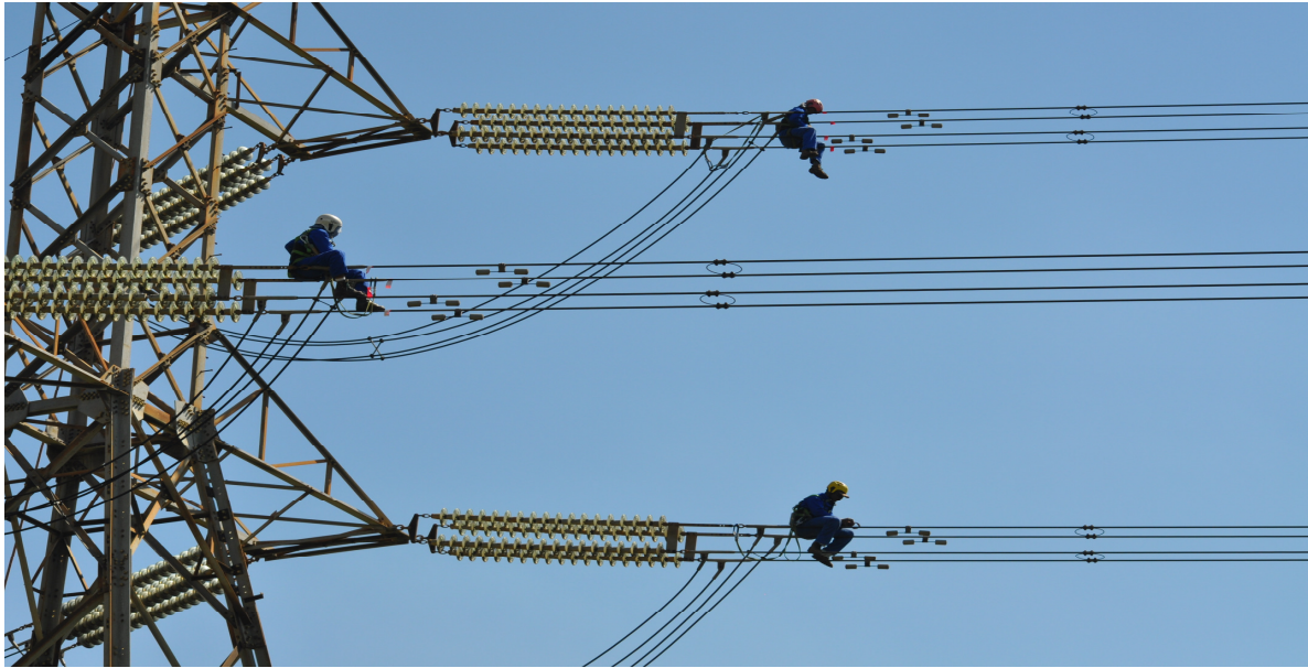
Figure 4.1.1: Workers installing temperature sensors onto conductors
