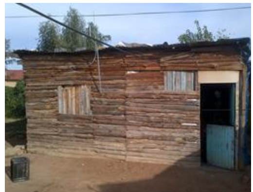
Figure 37: A timber backyard dwelling, typical in the case study
