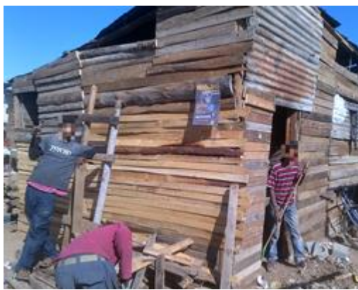
Figure 34: An informal backyard rental dwelling under construction
