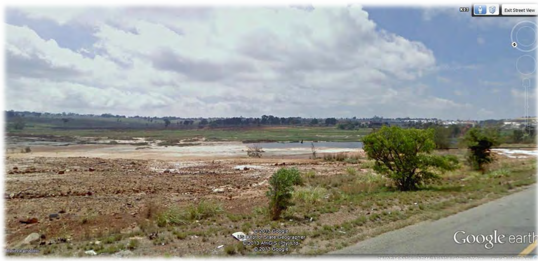
Photo E2.1: The Lancaster Dam (Note the tailings which form the base and shores of the dam)
