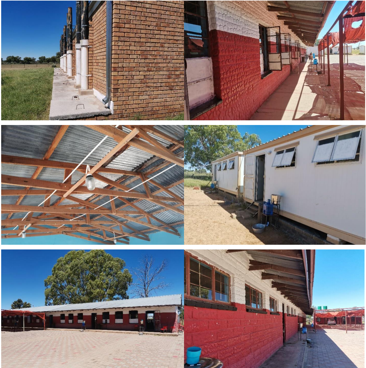
Gakgatsana Primary School – Site A Photo's (Source: Author's creation, 2022)
