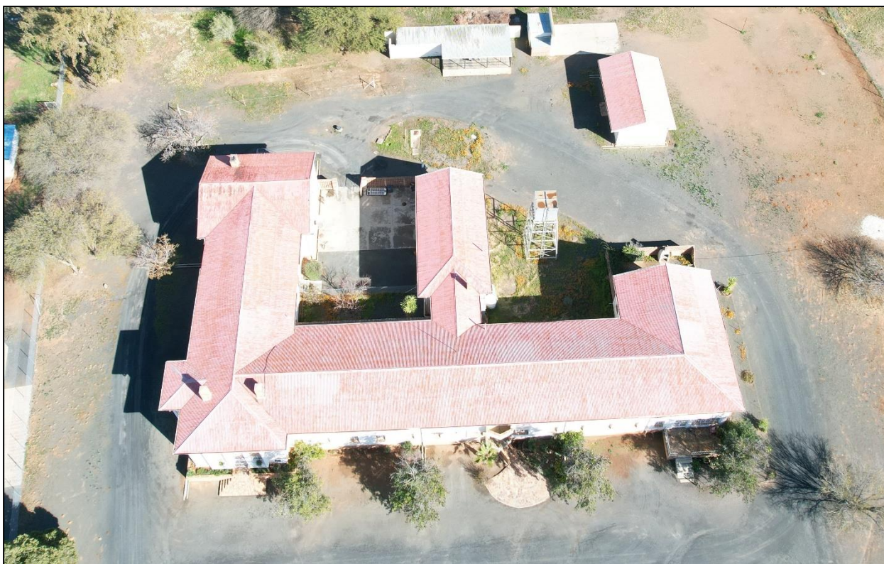
Figure 6-4: Drone Photo of Hoërskool Calvinia school
