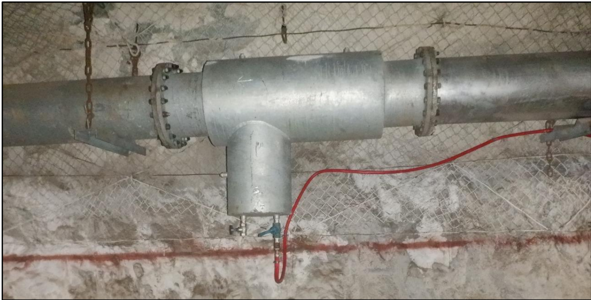
Figure 41: Installed water trap at 13L station
